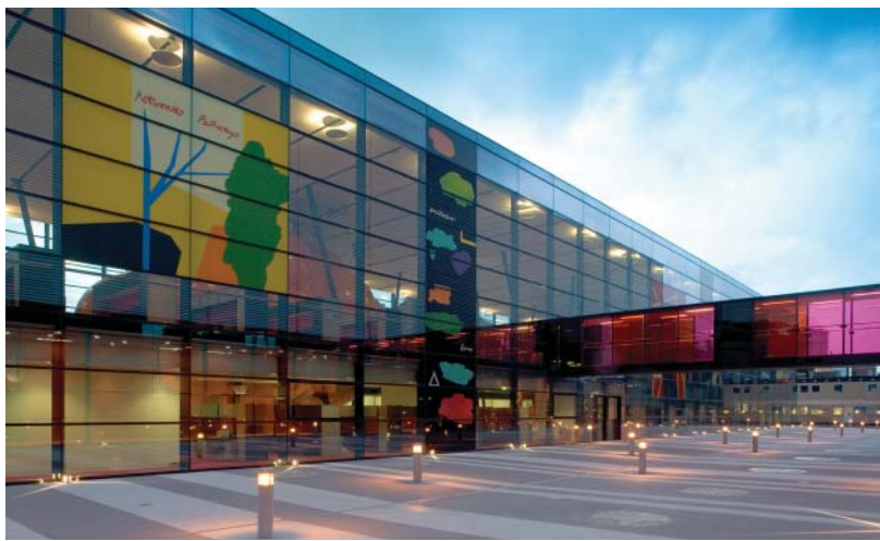
▲ Queen Mary, University of London The new building brings together many departments dispersed across a number of sites in a single collaborative research environment. The radical layout of the laboratory space encourages flexible working and breaks down knowledge silos. The workings of the building are made transparent and its supporting amenities are aimed at informing the public and children about modern medical research. Client: Queen Mary & Westfield College. Value: £34million. Completion: May 2005.
