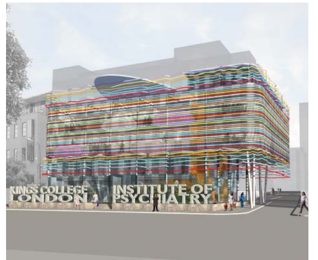
▲ King's College London, Institute of Psychiatry Alsoop are currently working with the IOP on proposals for the re-modelling of the main library and entrance building to the Denmark Hill campus. The project aims to break down some of the stigma attached to mental health.
